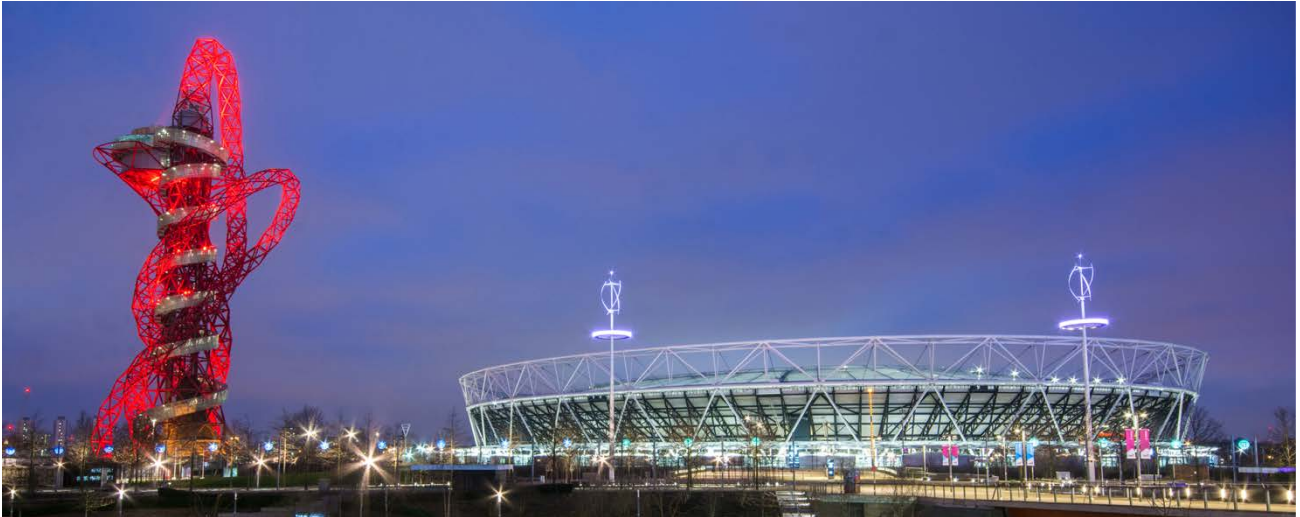
Olympic Stadium, London
