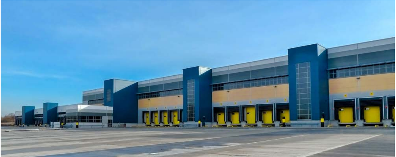
James Hall Distribution Centre
