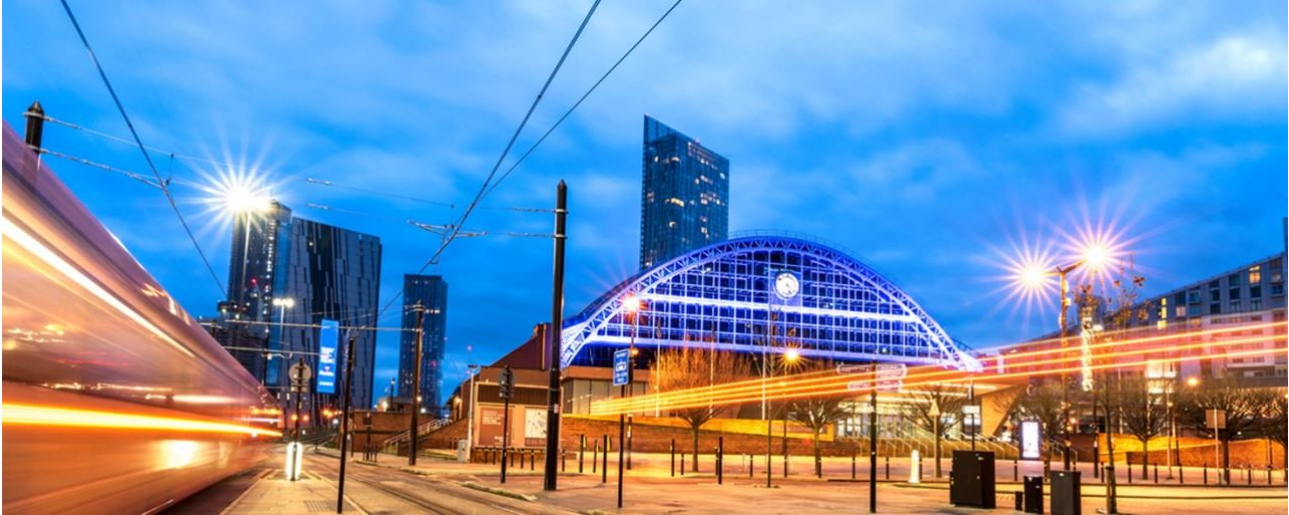
Manchester's Central Convention Complex
